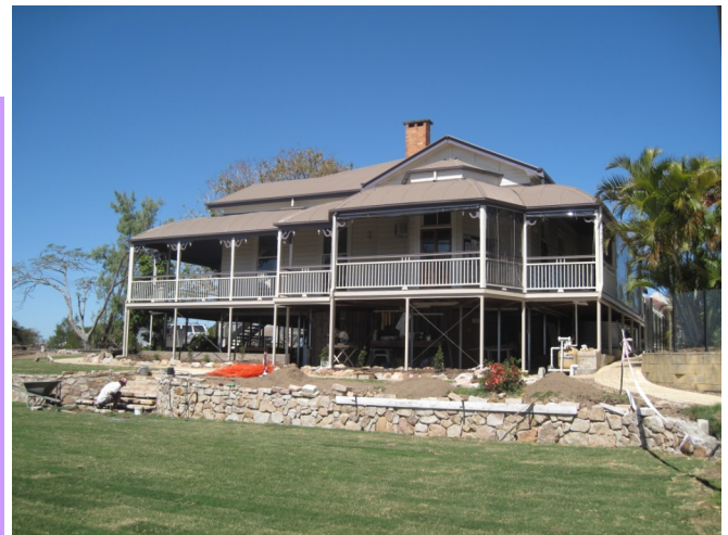
30 Lady Mary Terrace—final stage of renovation project, October 2009
